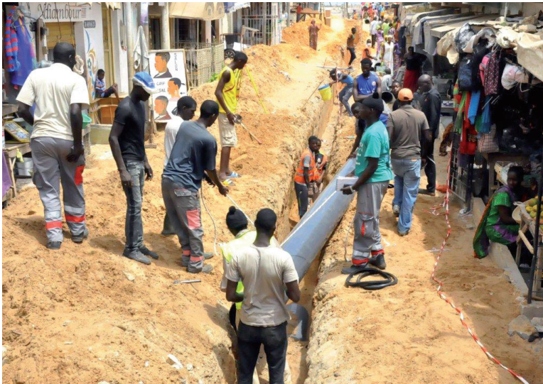
Ben Barak, Pikine, Dakar, Participatory infrastructure.
