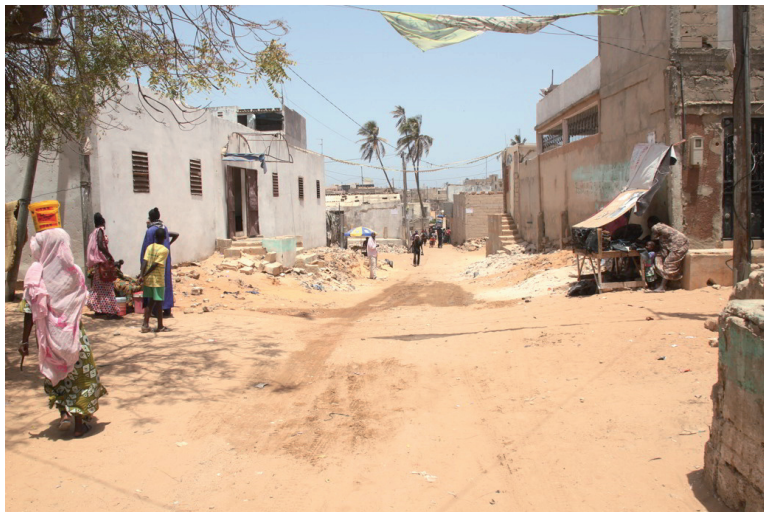
Main street to the market of Ben Barak suffering erosion in rainy seasons.
