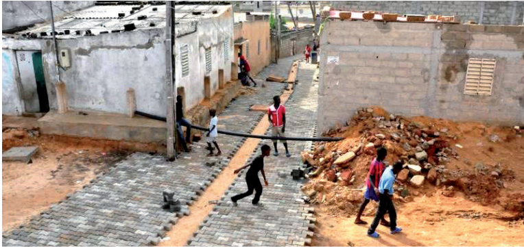
Main street to the market in construction.
